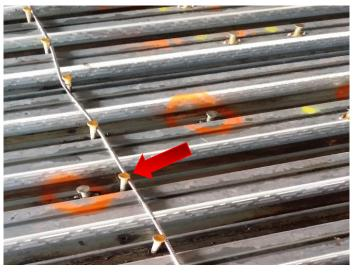
If installing temporary or permanent power in the slab on metal deck, make sure that the conduit is at least a 3" inches away from the studs in the deck.
